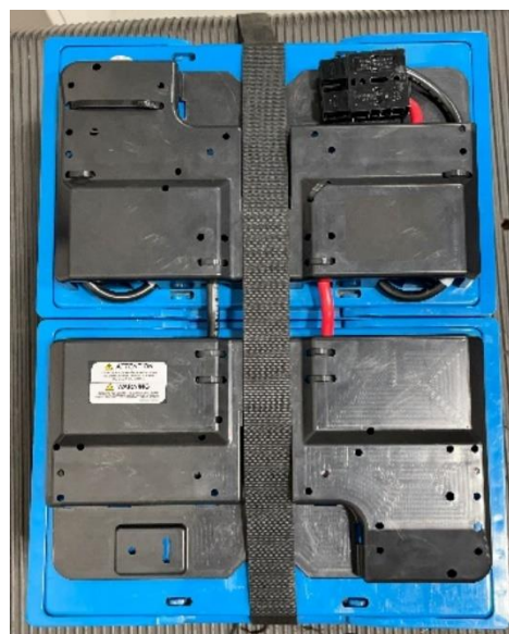
Cover installation as of October 1 st , 2021
